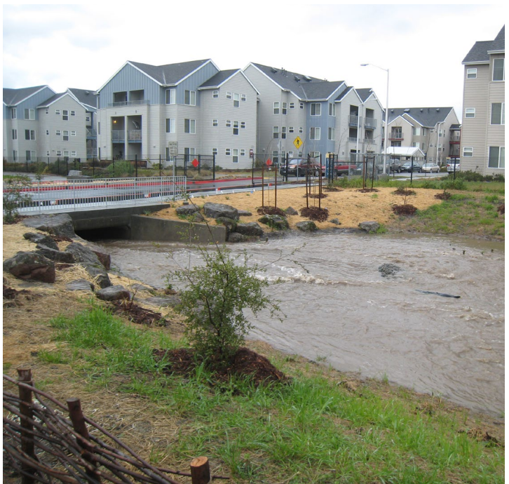
PHASE 3: Channel entering 6th street culvert during storm - 2.17.2011
