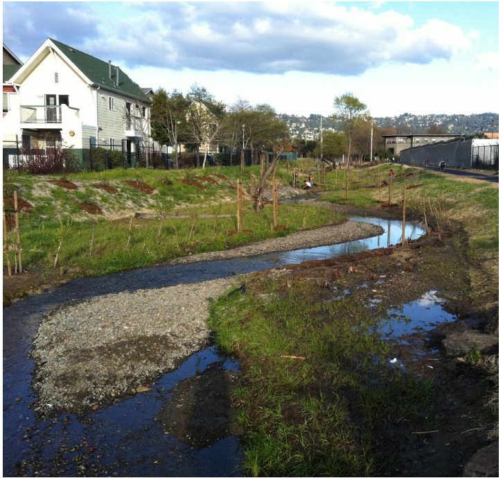
PHASE 3: Looking upstream from 6th Street after construction - 2.21.11
