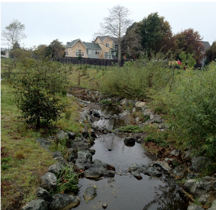
PHASE 3: Step pool channel below 8th Street Culvert - 10.24.11
