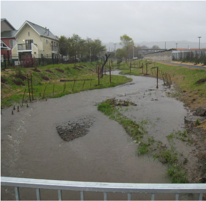
PHASE 3: Looking upstream from 6th street during high flows - 9.17.11
